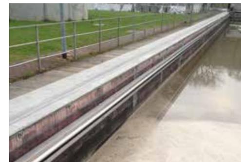
Longitudinal scraper, installed in the tank at Plauen sewage plant (Germany)
