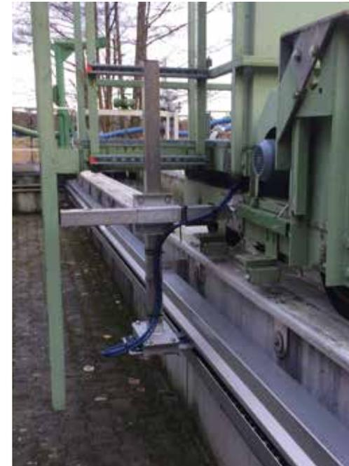
Sand traps with telescopic moving end arm
